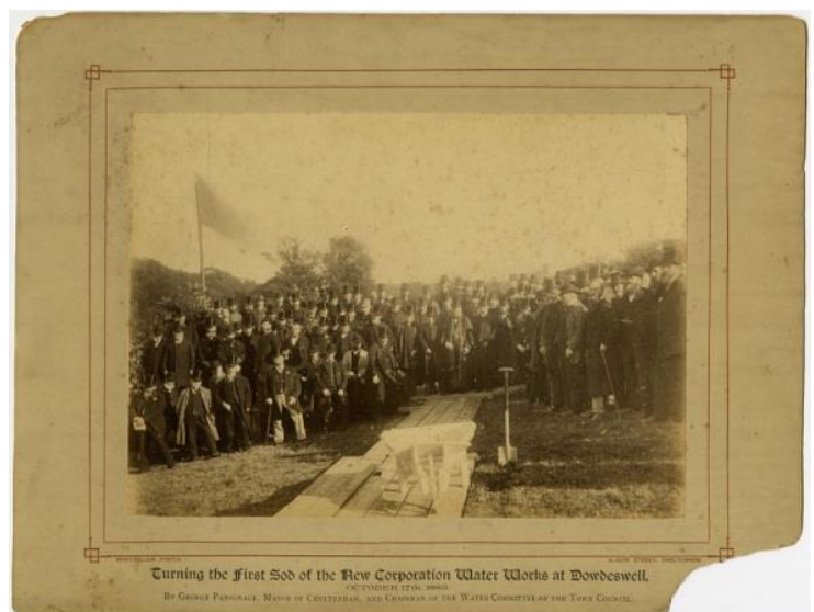
A photograph of the Mayor George Parsonage turning the first sod of the New Corporation Water Works at Dowdeswell
